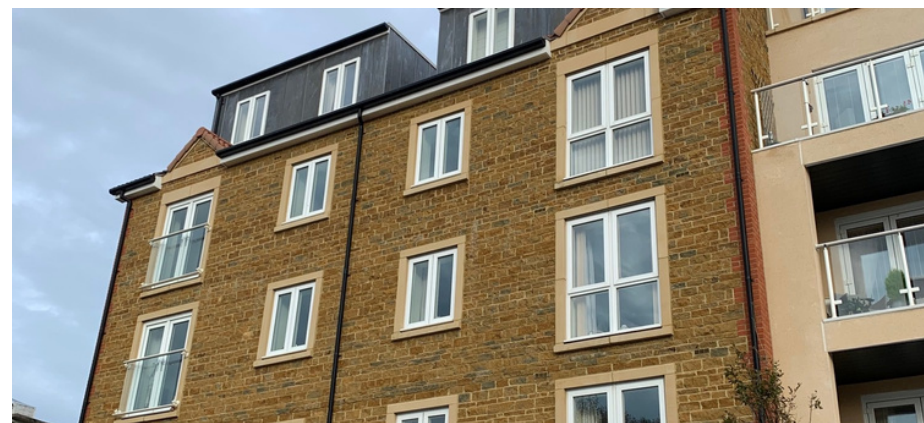
Image 1. Exterior of one of the buildings surveyed
